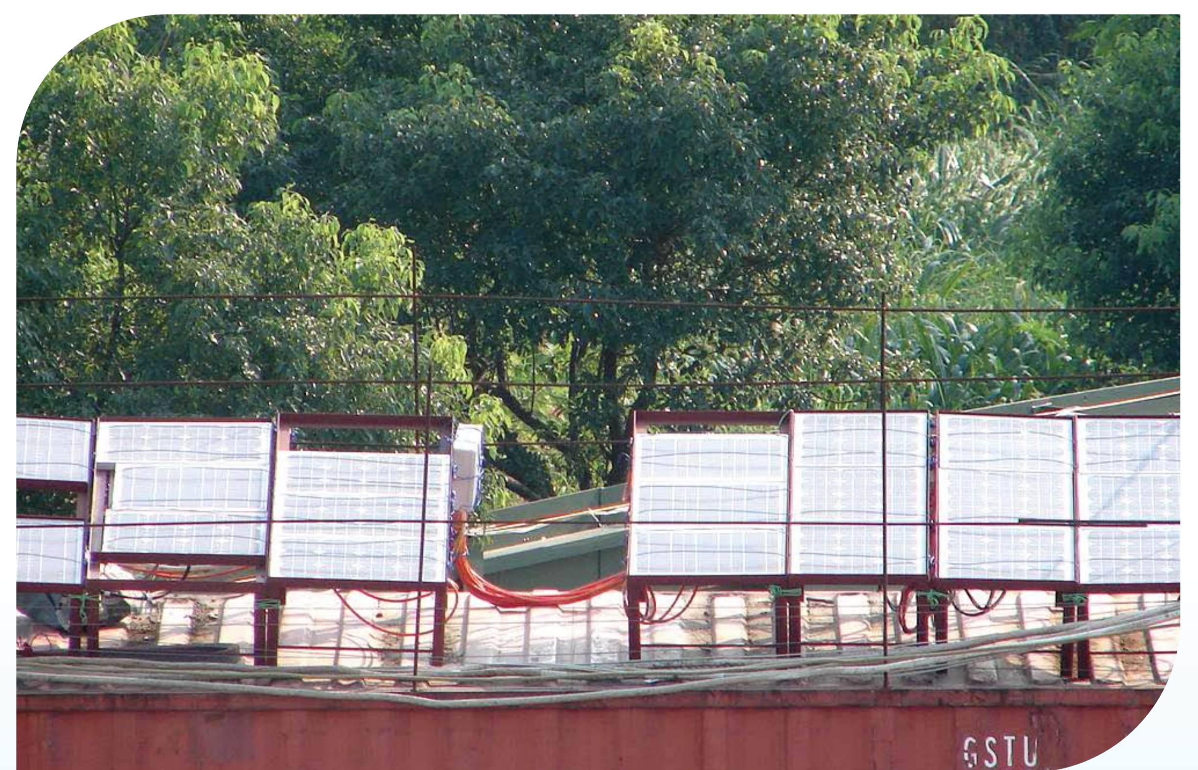
太陽能發電 Solar Power Energy Panel
