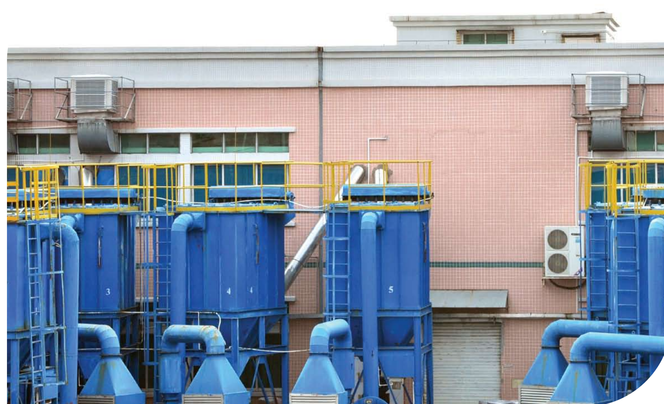
環保設施 - 廢粉處理系統 Environmental facility - Toner treatment system
