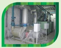
採用中央真空及鼓風系統,節約能源和減少對空調的損耗。 Central vacuum and air-blowing system not only offers better efficiency but also lowers air-conditioning loading.
