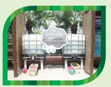
在場內不同位置設置雨水收集儲水缸,用作灌溉場內植物。 Rainwater collection systems placed at numerous locations allow the stored water to be used for irrigation.
