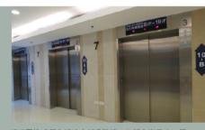
透過更換或優化超過十部升降機・包括安裝發光二極 管燈、可變壓控制器和電源再生功能,以節省能源。 Replacing or upgrading over 10 lifts by installing LED lights, variable voltage controller and power regenerative functions to
