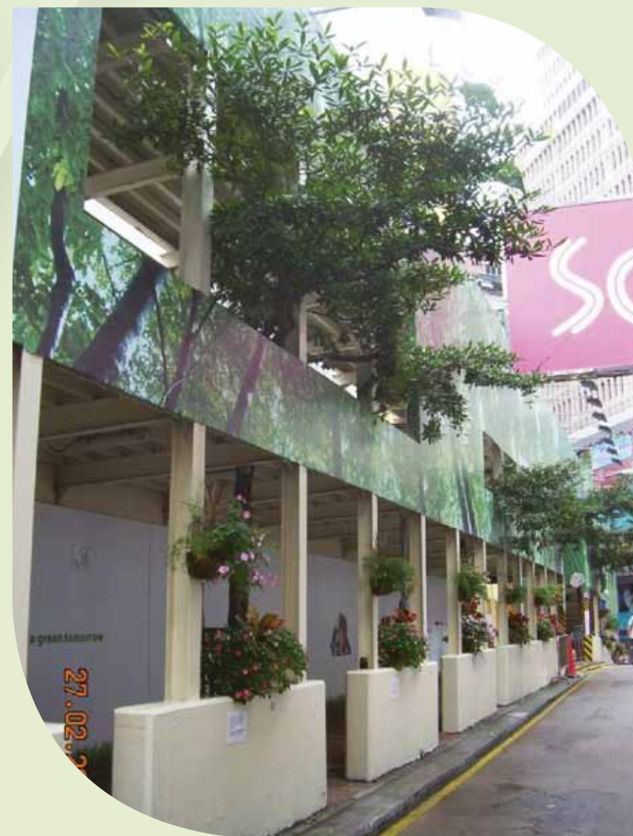
建立綠化圍板 Establishment of Green Hoarding
