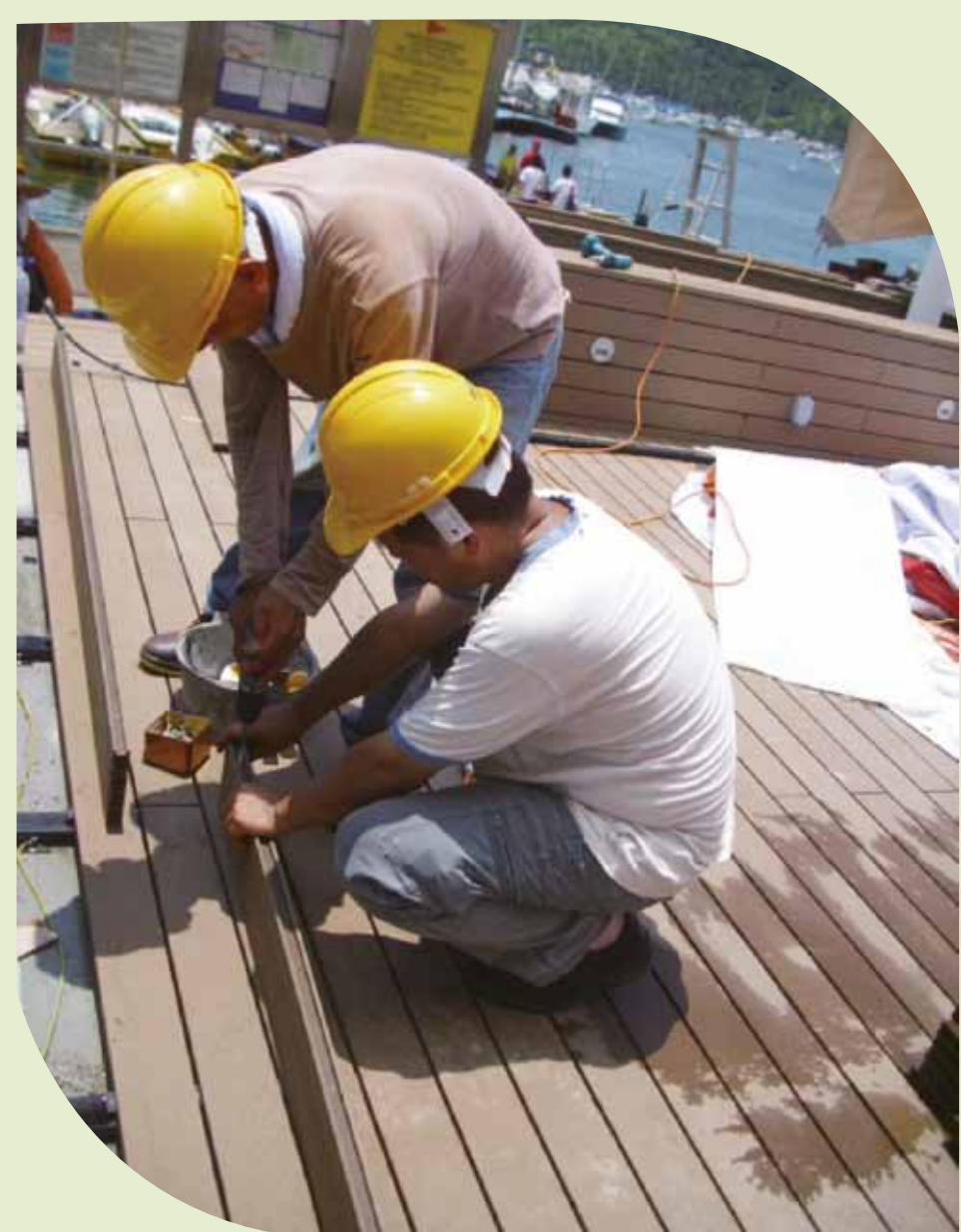
採用循環再用物料代替木材製作甲板 Replacing wood with recycled material for decking
