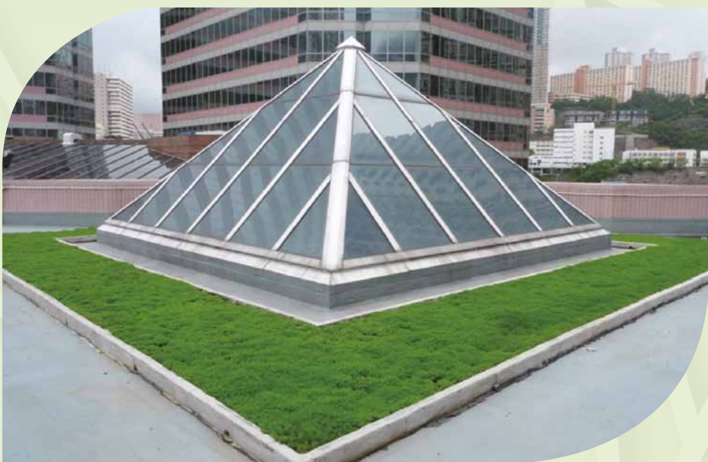
於噴泉廣場及5樓天台種植有助降低室溫的佛甲草地 Fijian Grass fields at Open Piazza and L5 Roof tops help to lower the room temperature underneath
