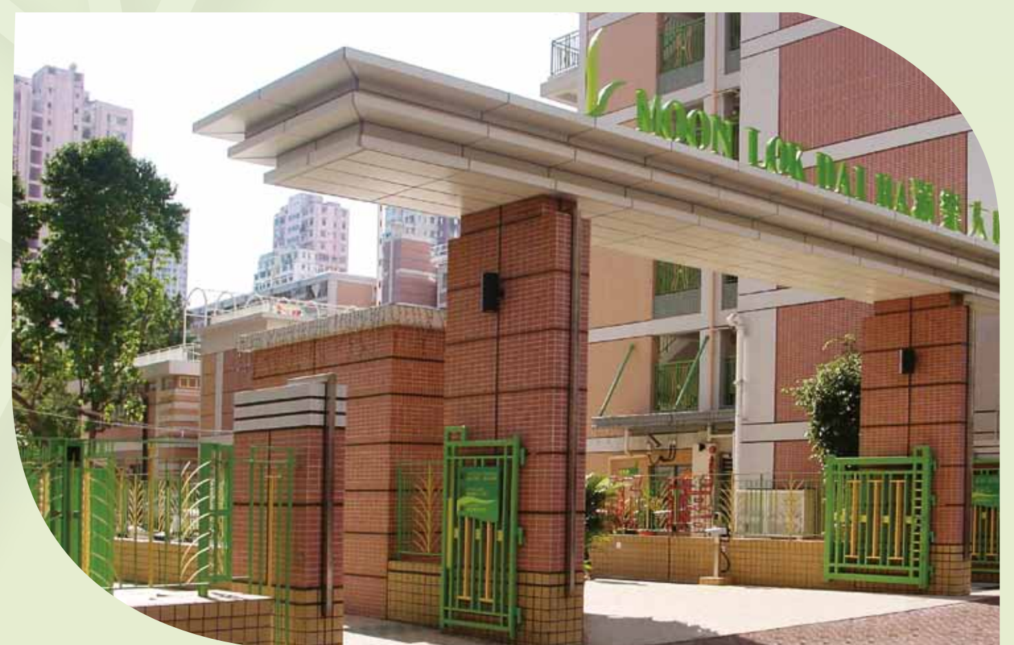
以復修取代重建，可減少建築及拆卸所產生的廢料。 滿樂大廈的復修工程是最佳例子。 Instead of redevelopment, rehabilitation would produce less construction and demolition waste. The rehabilitation of Moon Lok Dai Ha is the best example.
