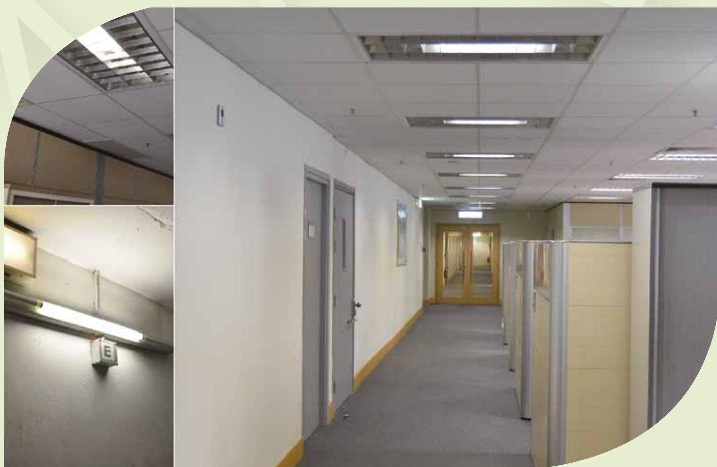
透過於大樓更換節能燈具，節省耗電最少百分之六十。 Replacement of lighting with energy saving models in the whole premises, more than 60% of electricity is saved.
