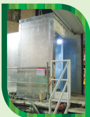
雙重門入口是隔音罩其中一個重要組件。用隔音板組成雙重門入口，目的是確保當有需要進出隔音罩時，亦不會洩漏噪音。 Double door entrance is an important component for the noise enclosure. The double door entrance is made up of noise panels aiming to ensure that noise will not be leaked out from the noise enclosure during access.
