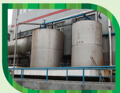
蒸汽回收再用 Reuse the condensate steam
