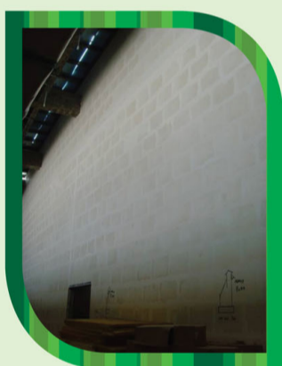
無須鐵網、門樑及鋼鐵支架，減少使用額外材料進行安裝，降低能耗。 No supporting materials such as metal mesh, lintel and steel stiffener are required.
