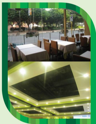
使用LED燈及T5光管，在貴賓區採用自然光。 LED lamp and T5 Fluorescent lamp in the restaurant and natural light in VIP area.
