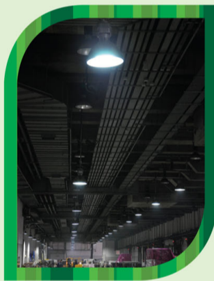
將倉庫逾600套鹵素燈更換成電磁感應照明燈及節能日光燈，節省的電量多達百分之五十。 Over 600 sets of Hi-Bay lights in warehouses were replaced by energy-efficient induction lamps and fluorescent light fittings saving more than 50% of energy.
