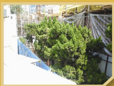
施工期間使用膠布及圍板保護樹木，亦在圍板加設開口以利通風。 During construction, plastic sheets and hoarding were used to protect trees. Additional openings at tree hoardings were used to improve ventilation.
