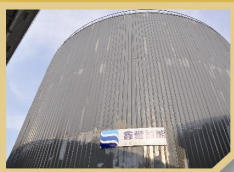
水蓄冷空調可節省運行費用達30-60%及減輕用電量。 Water Storage Air Conditioning reduces the operating cost by 30-60% and the electricity consumption.
