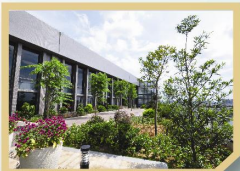
持續空中花園能淨化空氣，隔熱保溫。 Green wall and roof garden help purify air and reduce indoor temperature.
