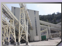
完全密封的石場破碎機以及混凝土攪拌機和噴霧乾燥機加以隔離，確保符合環保標準。 The fully enclosed quarry crushing plant and the concrete batching plants isolate dust and noise emissions from their sources ensuring that the environmental standard is met.
