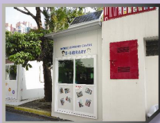
設置太陽能板，讓學生了解再生能源的技術。 A solar panel has been installed to educate students about renewable energy.
