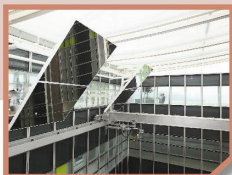
ETFE 天窗及太陽光反射導入系統以減省用電。 ETFE roof and reflective mirror to reduce energy.
