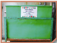
收集冷氣系統的冷凝水，用來洗車、掃地和灌溉植物。 Condensed water from air-conditioning system is collected for cleaning, planting and car washing.
