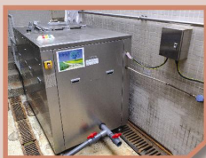
廚餘機可每天可處理300公斤廚餘。 The food waste decomposer handles 300kg of food waste daily.
