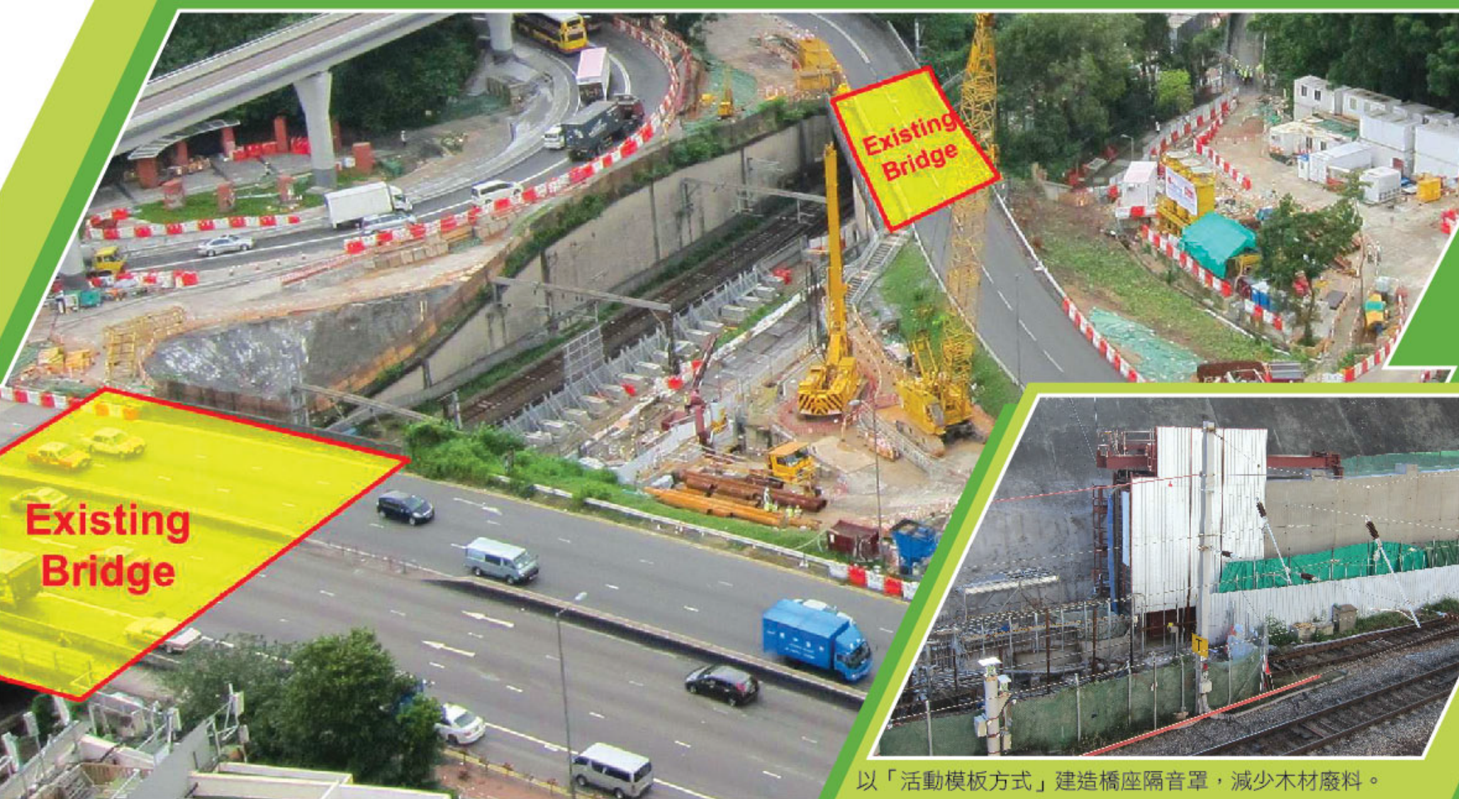
利用循環再用的貨櫃及廢鋼建造「組合式灌漿台」平台。 Building "Modular Grouting Platform" with recycled containers and scrap steels.
