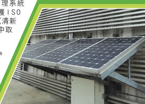
安裝太陽能電池板,為天台花園的燈柱供電。 Installing solar panels to supply electricity for the lamp posts at roof garden.
