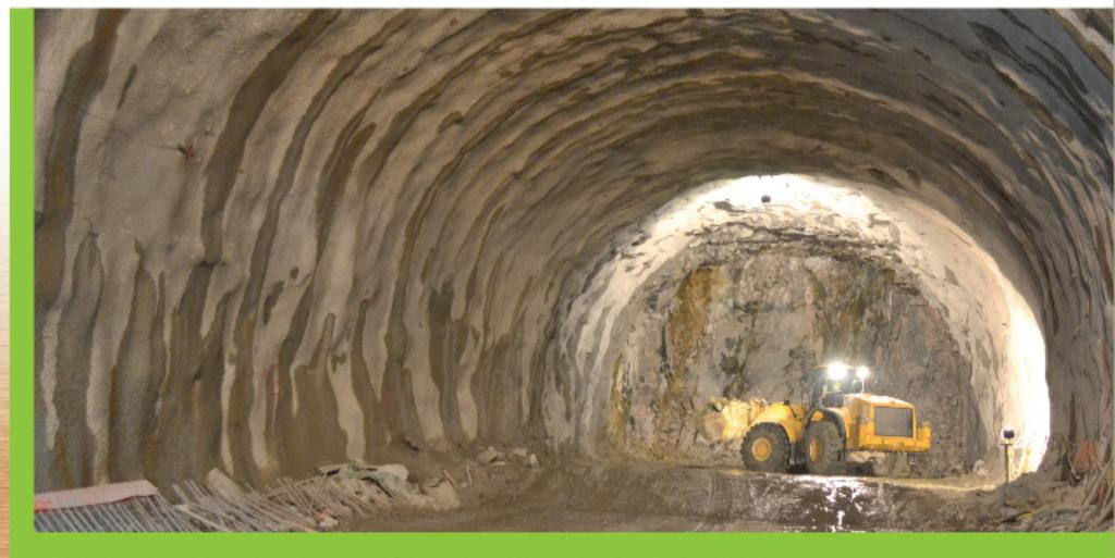
修改隧道管道設計從而縮減隧道橫切面積,減少挖掘量。 Altering tunnel design to reduce the size of tunnel cross section and excavation volume.
