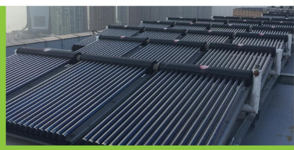
在天台安裝超過二百套太陽能板/管收集熱能,以加熱用水。 Installing over 200 sets of solar panels / tubes on the rooftop to collect solar energy for water heating.
