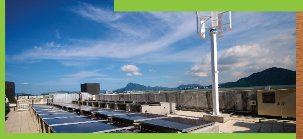
天台裝有太陽能板及一台風力發電機,提供部份電力供大樓使用。 Installing solar panels and a wind turbine on the roof to support part of the electricity for the main building.
